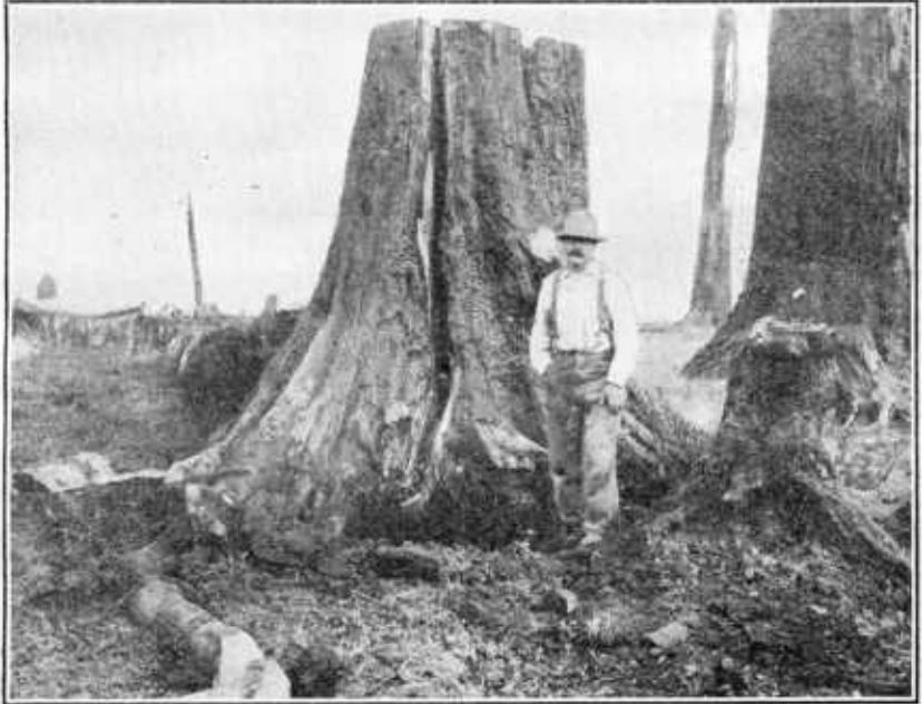
FIG. 5.—This stump was cracked for burning as described under the Northwest method. Six and one-half pounds of dynamite were required.
